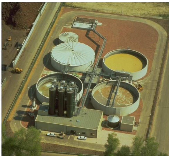
Figure 16.21 (A) IC installation for treatment of @ and (B) EGSB installation for treatment of (photo: Paques B.V. and Biothane B.V. respectively)
