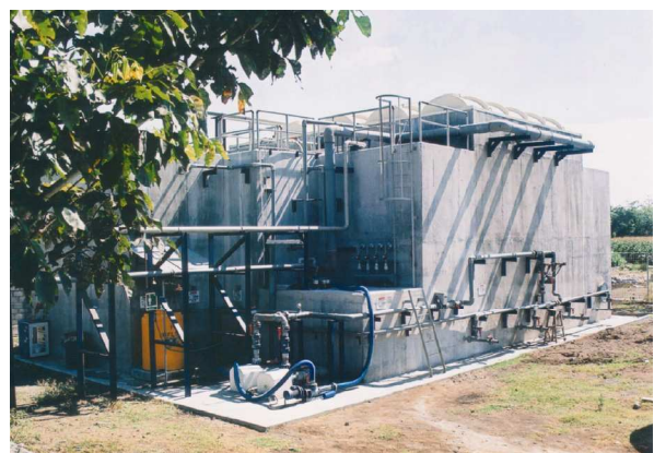
Figure 16.18 UASB installations for treatment of (A) agro-industrial and (B) dairy wastewater in Indonesia (photo: Paques B.V. and Biothane B.V. respectively)
